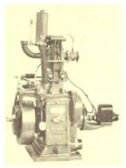
Early CFR engine (credit: CFR Inc.)
